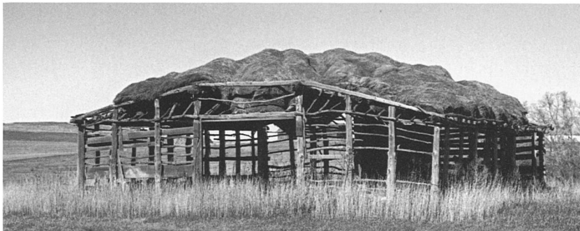
Fig. 8. Wallace Osadchuk cattle barn. The barn originally had mounds of straw packed loosely around the earthfast frame. (Author)
